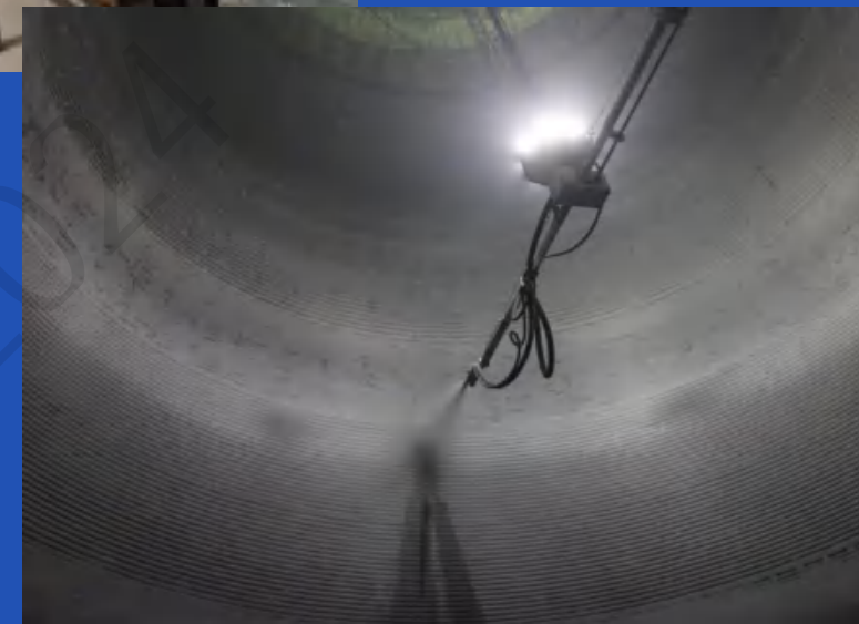
高炉内衬喷注修复 Shotcrete lining for blast furnace relining
