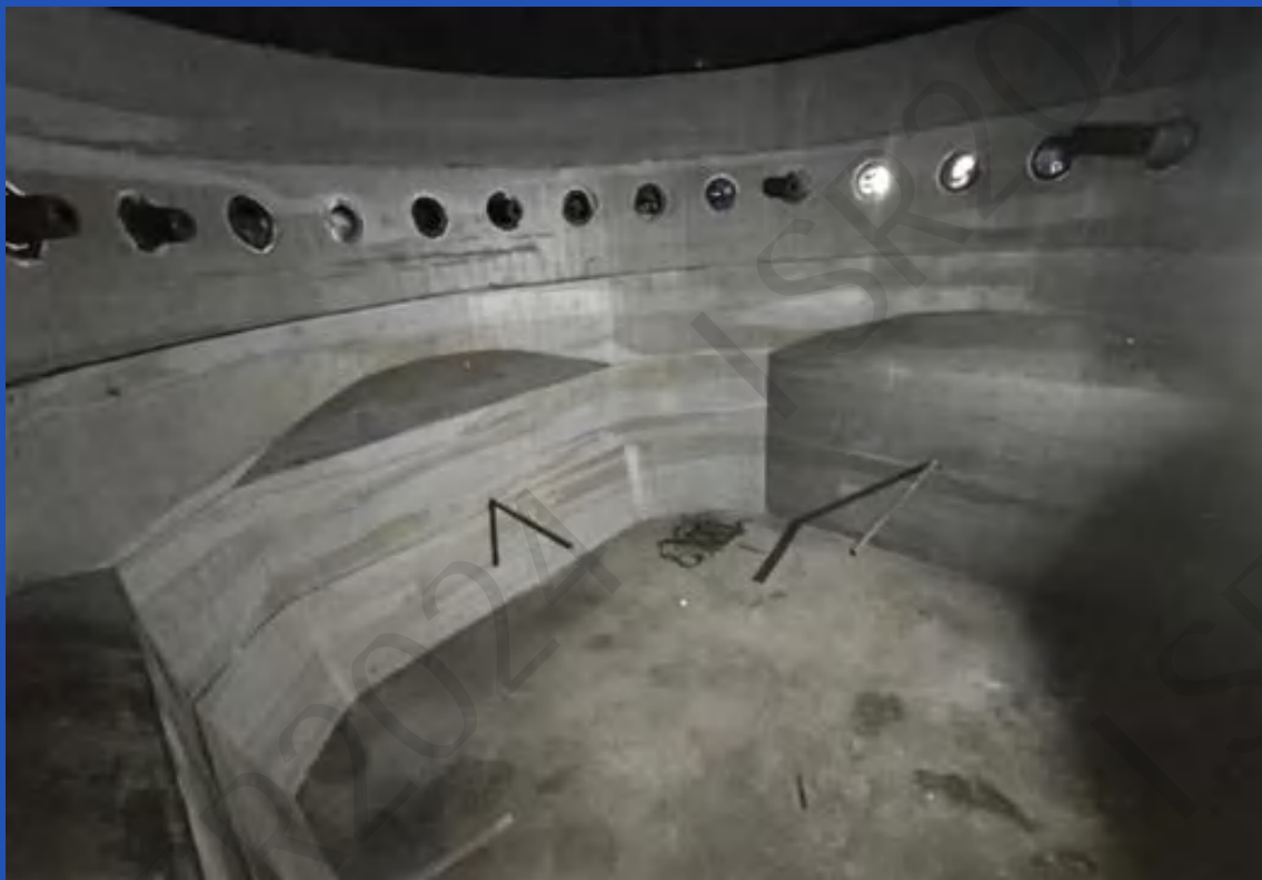
炉缸整体浇注 Monolithic hearth casting of BF
